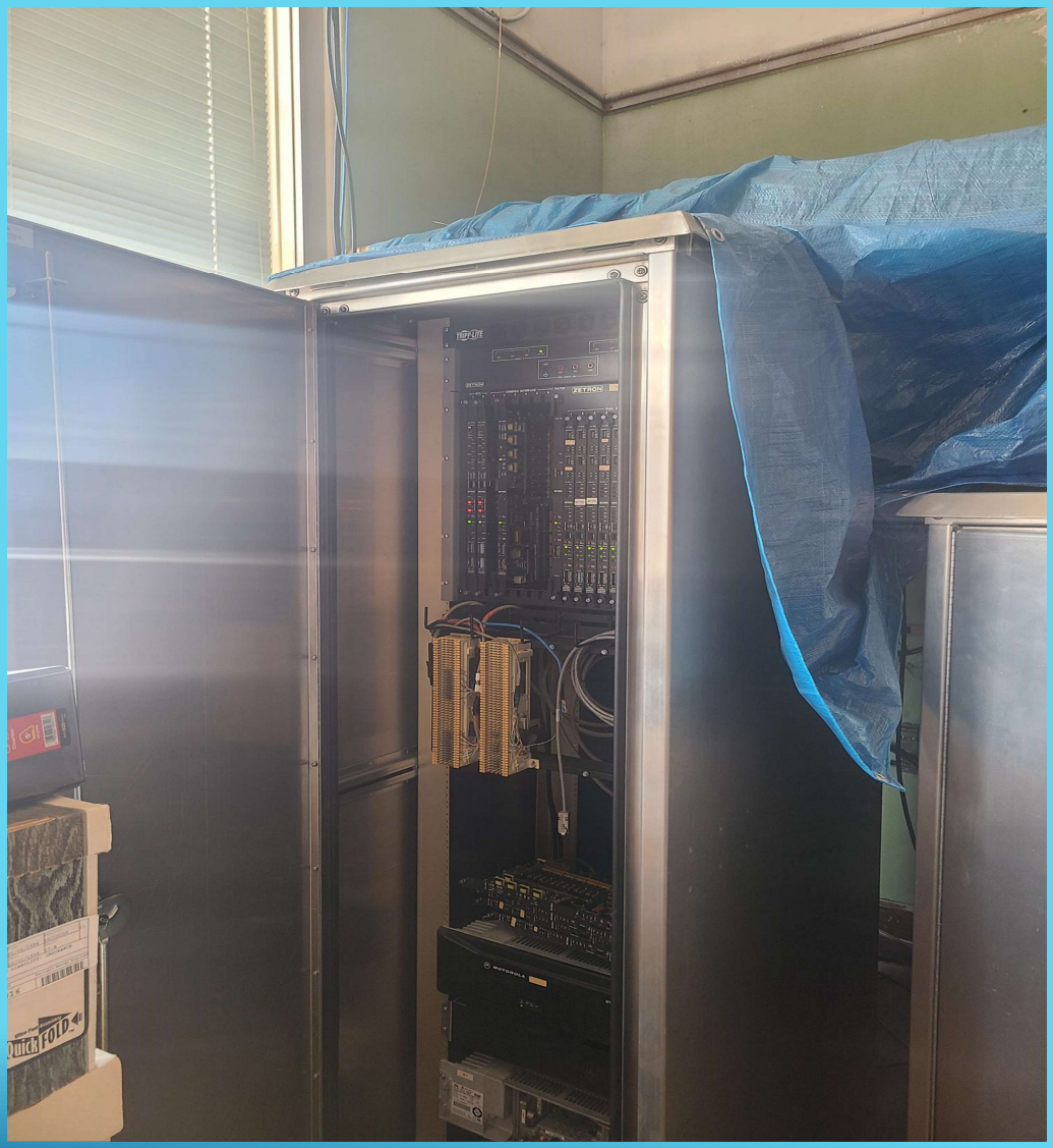
Damaged radio equipment on 2 nd floor.
