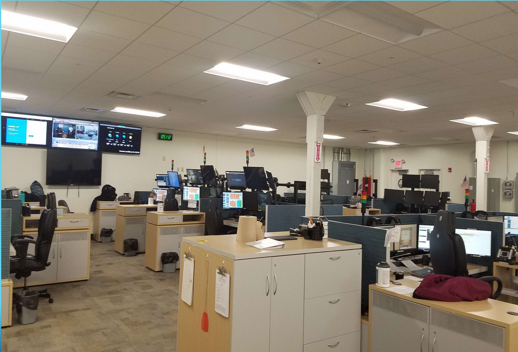
Cape May County Communications Center, Main Radio Room.
