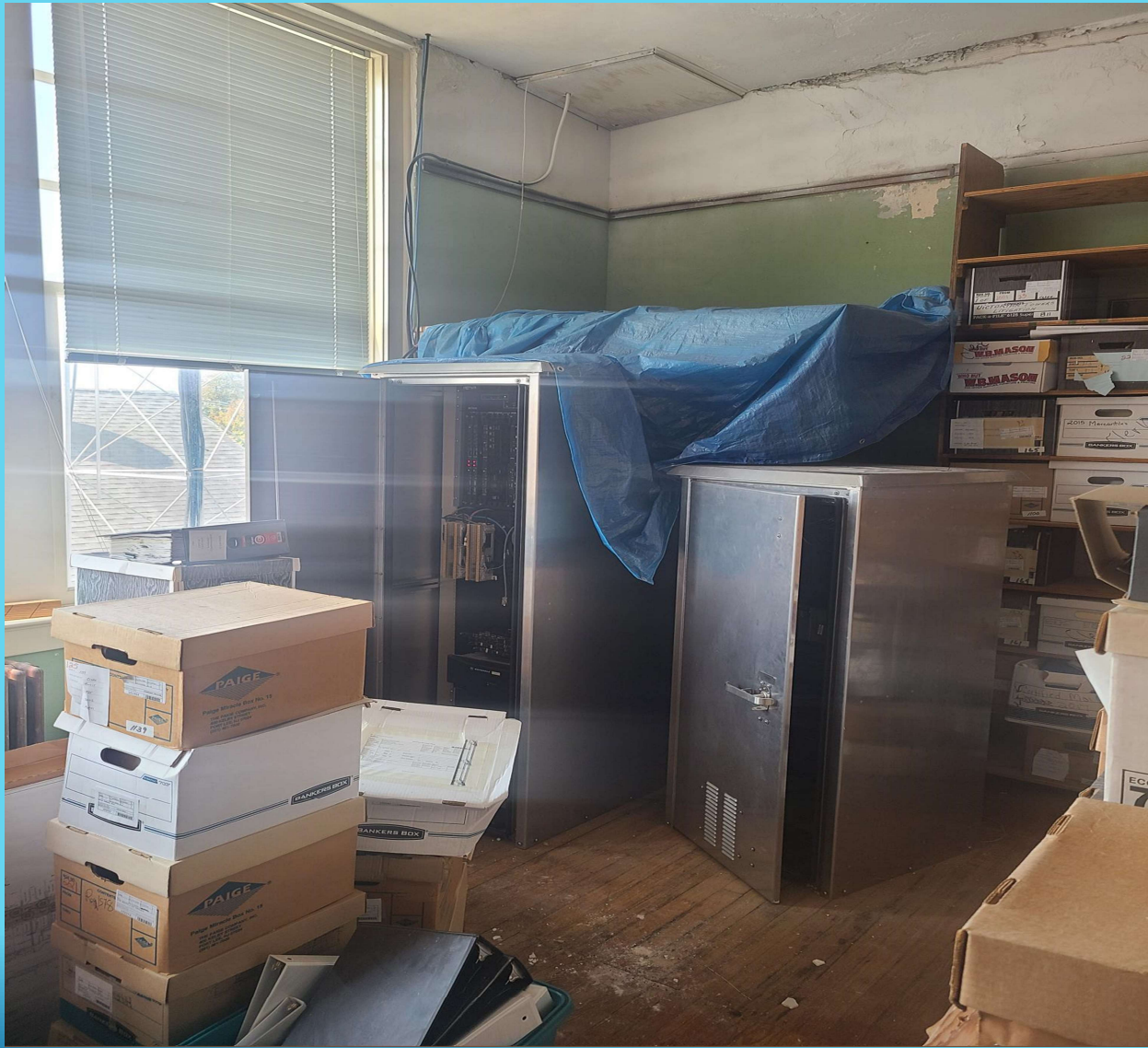
Damaged radio equipment on 2 nd floor.
